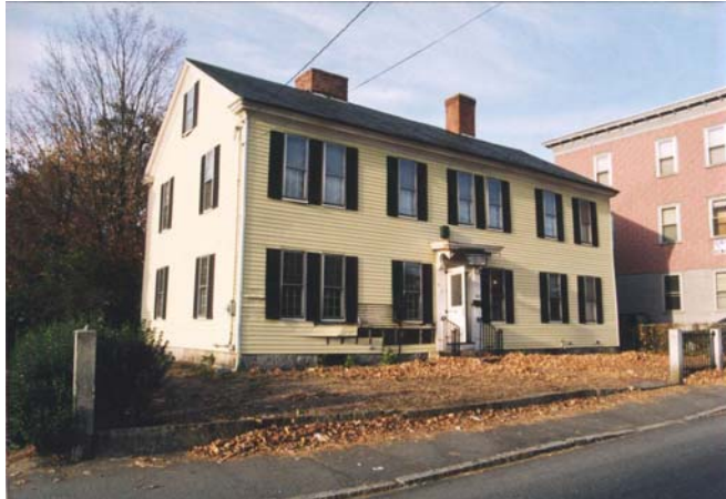
Spalding House – after removal of aluminum siding
